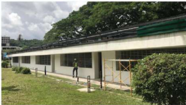
PDRF Emergency Operations Center Building (October 12, 2017)
